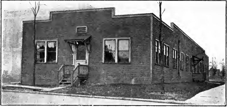
Headquarters Building of the Development Division, Nela Park
